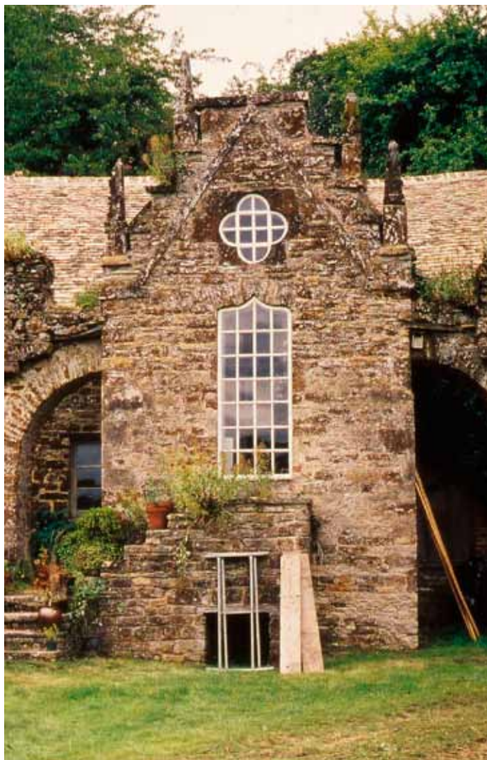
Fig. 3 The Mill, gothicized by Kent.
